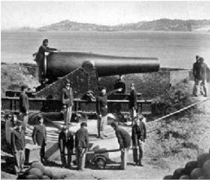
The huge 20 inch Rodman cannons were only fired a few times for practice. In reality, most coastal defense fortifications eventually used the 10-inch or 15-inch Rodman cannons. Alcatraz originally had 10-inch Columbiad cannons but in 1864 the island received the better constructed Rodman 15-inch cannons.
