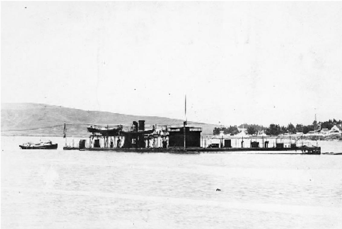
The *Comanche* off of Mare Island, 1898. Its steel sides were 5 1/2 inches thick, the sides of the turret were 11 in. thick, with an inch of iron on its deck. It had two 15 inch smoothbore cannons in its turret. Its two boilers provided steam for propulsion and for moving the spindle which rotated the turret
